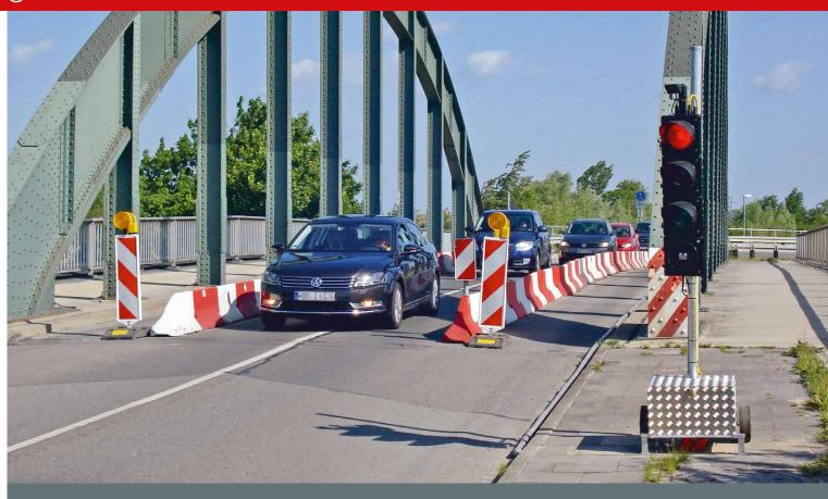
MPB 4400 – radio-controlled signal system, vehicle-actuated for alternating one-way traffic, can be extended for crossroads.
